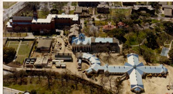
Construction aerial view of The Village February 28, 1988
